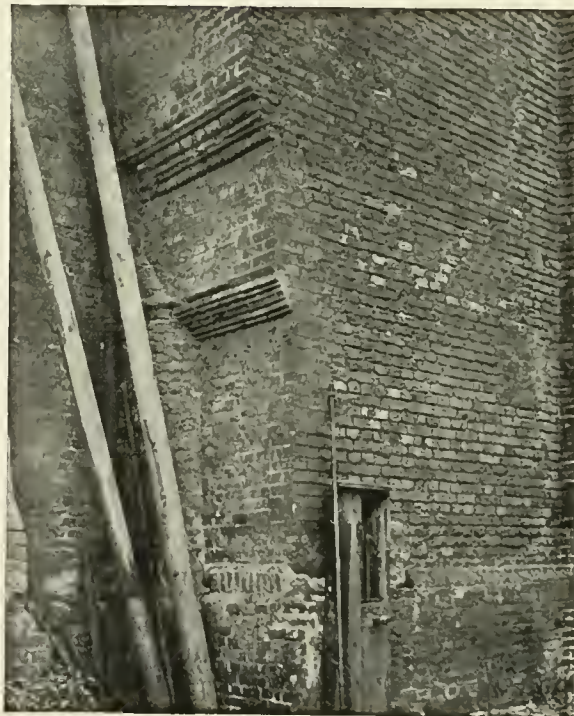
(a) ARCH UNDER CHIMNEY-STACK
